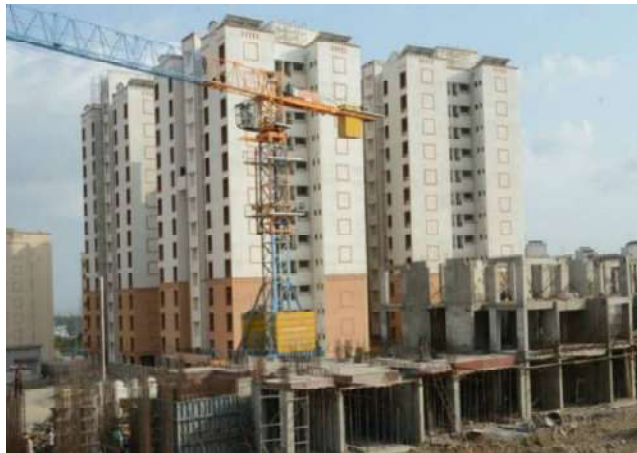
1. AHP Houses in Pune, Maharashtra using Precast Construction Technology
