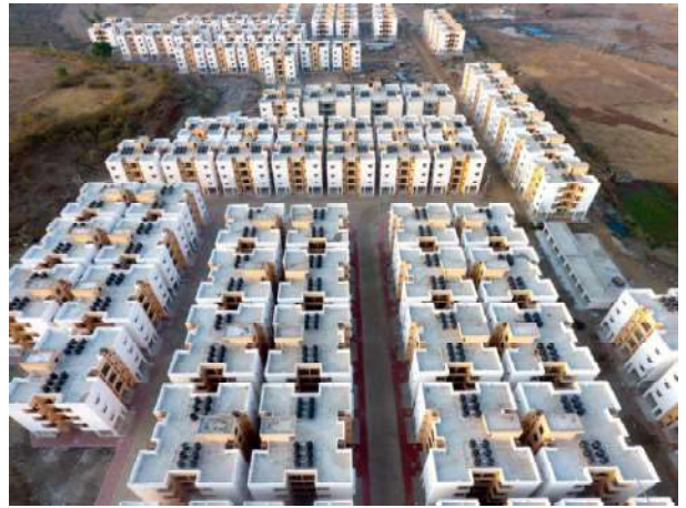
4. PMAY(U) Project in Chindwara, Madhya Pradesh
