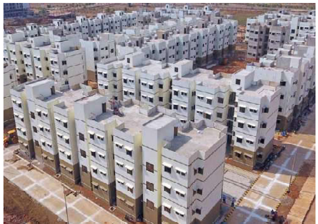
2. AHP Houses in Atal Nagar, Chhattisgarh using Precast Construction Technology
