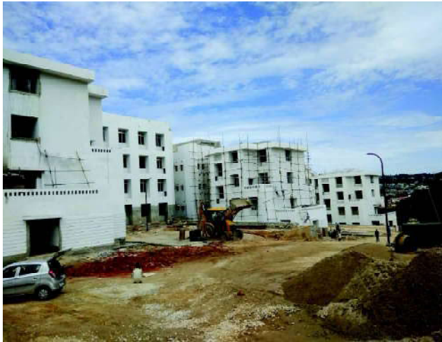
Construction of Office cum Laboratory Complex including Regional Training Institute of Geological Survey of India, NER at Shillong
