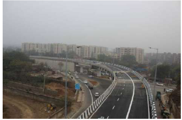
Newly constructed Flyover and Underpass between Northern Mahipalpur Bypass Road and Airport Road, Delhi
