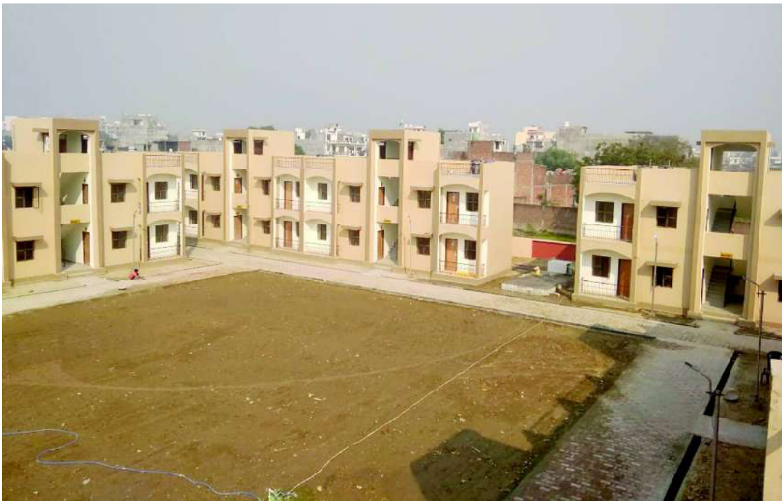
Demonstration Houses (40 DUs) constructed using Stay in Place EPS based double walled panel System by BMTPC at Aurangabad Jagir, Lucknow, Uttar Pradesh
