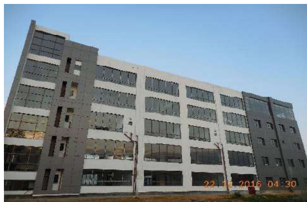
New Administrative Building at NIT Silchar
