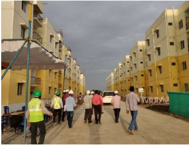
3. AHP houses in Andhra Pradesh using Monolithic Concrete Construction
