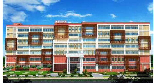
Proposed Redevelopment of Govt. of India Press at Minto Road, New Delhi
