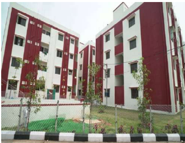
7. PMAY(U) Project in Telangana
